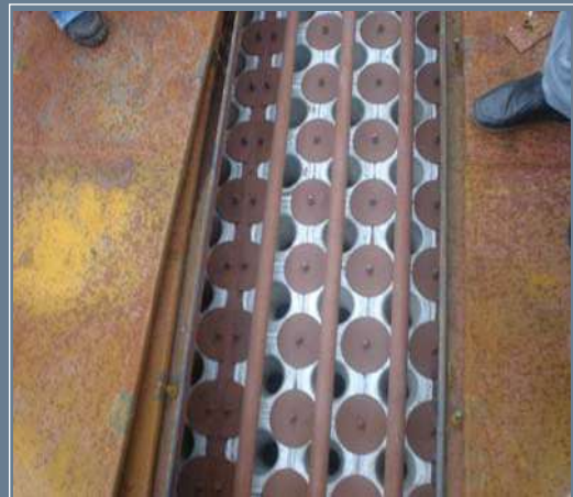
Typical bag filter arrangement
