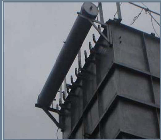
Compressed air piping for bag house
